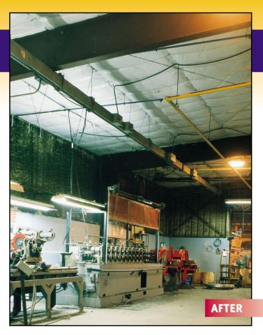
The fiberglass blanket shall be fastened to the purlin flanges and supported every two feet (2 ft.) by a white aluminum strap formed over the wrapped purlin flange. The strap shall extend transversely to the adjoining purlin where it interconnects with a previously installed strap to form a generally aligned, end-to-end relationship. All straps shall be screwed to the bottom side of the purlins at each point of attachment.
